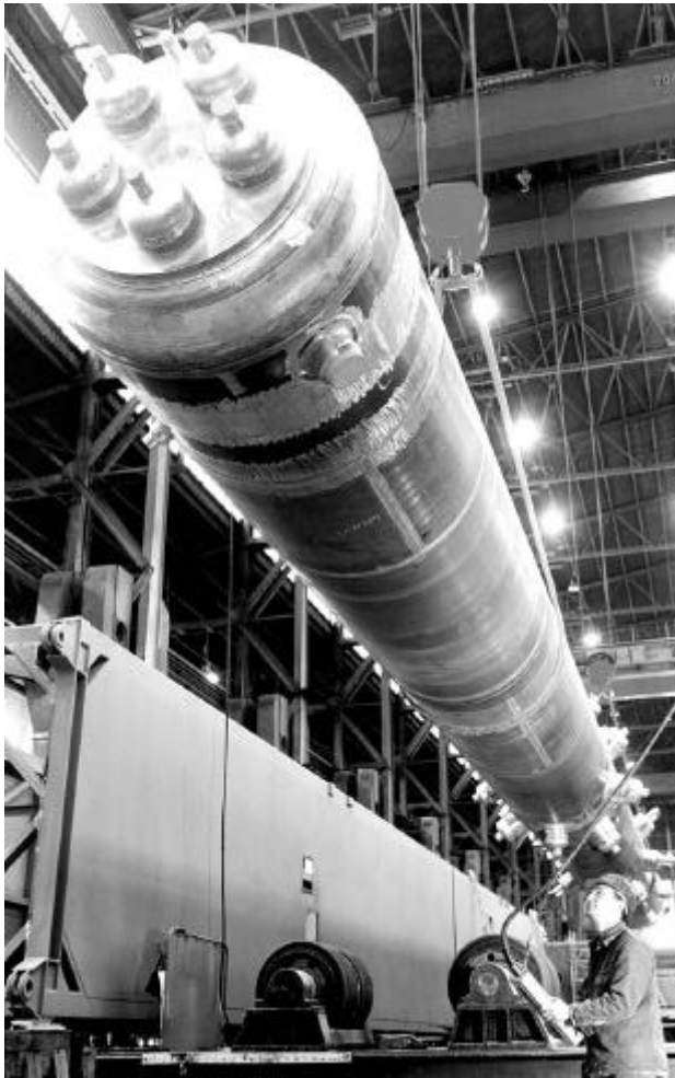
Fig.9: SWHE Installation into Cold Box
