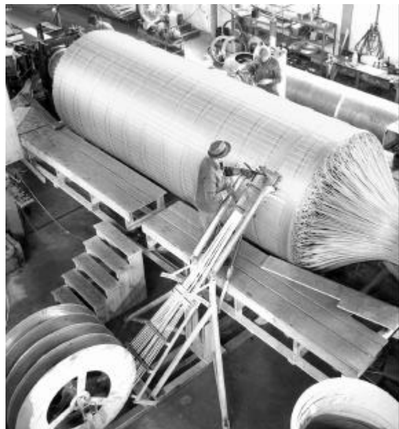
Fig.2: Tube Bundle Winding around 1950
