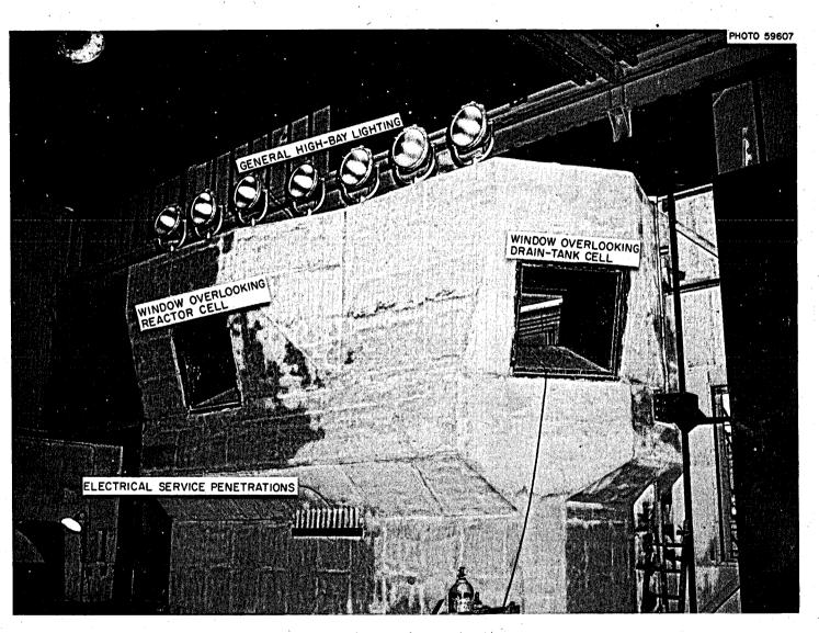
Fig. 2. High-Bay Side of Remote-Maintenance Control Room.
