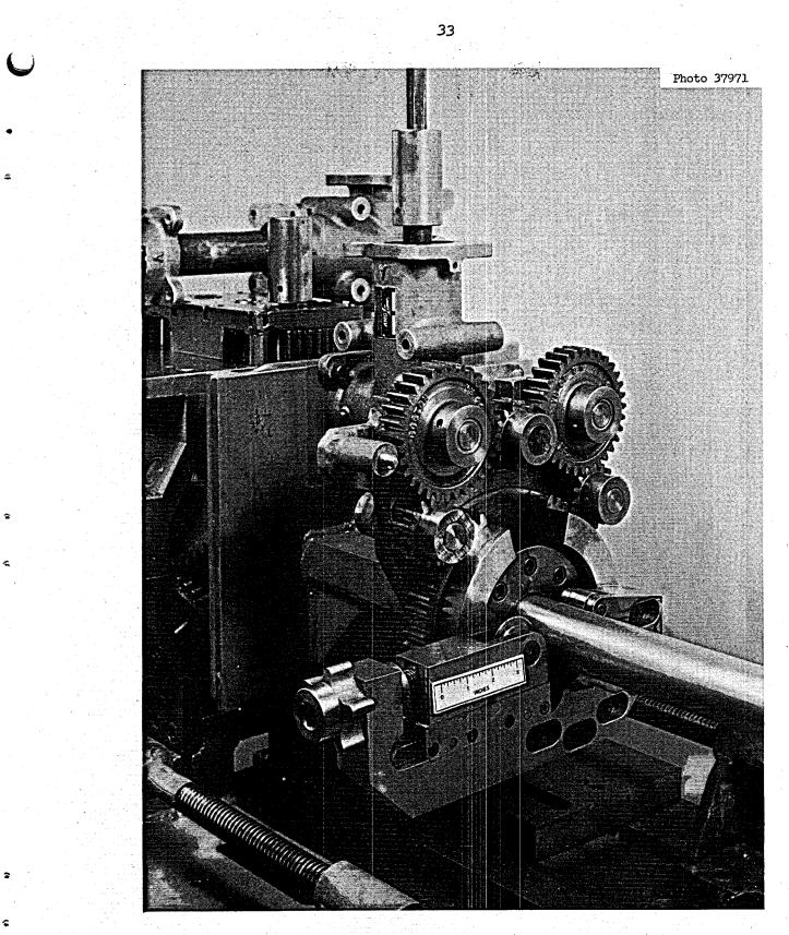
Fig. 19. Pipe Cutter for Remote Brazing.
