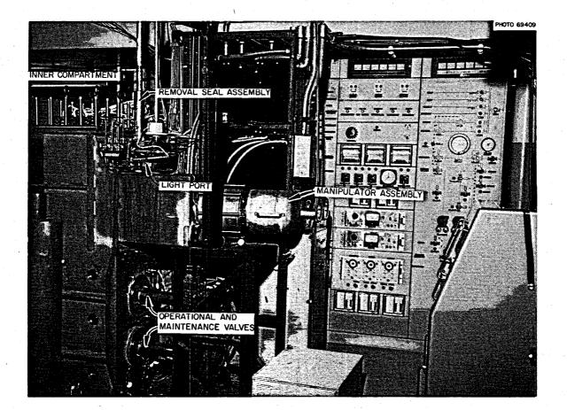
Fig. 23. Sampler-Enricher Installation Prior to Erecting Shielding.
