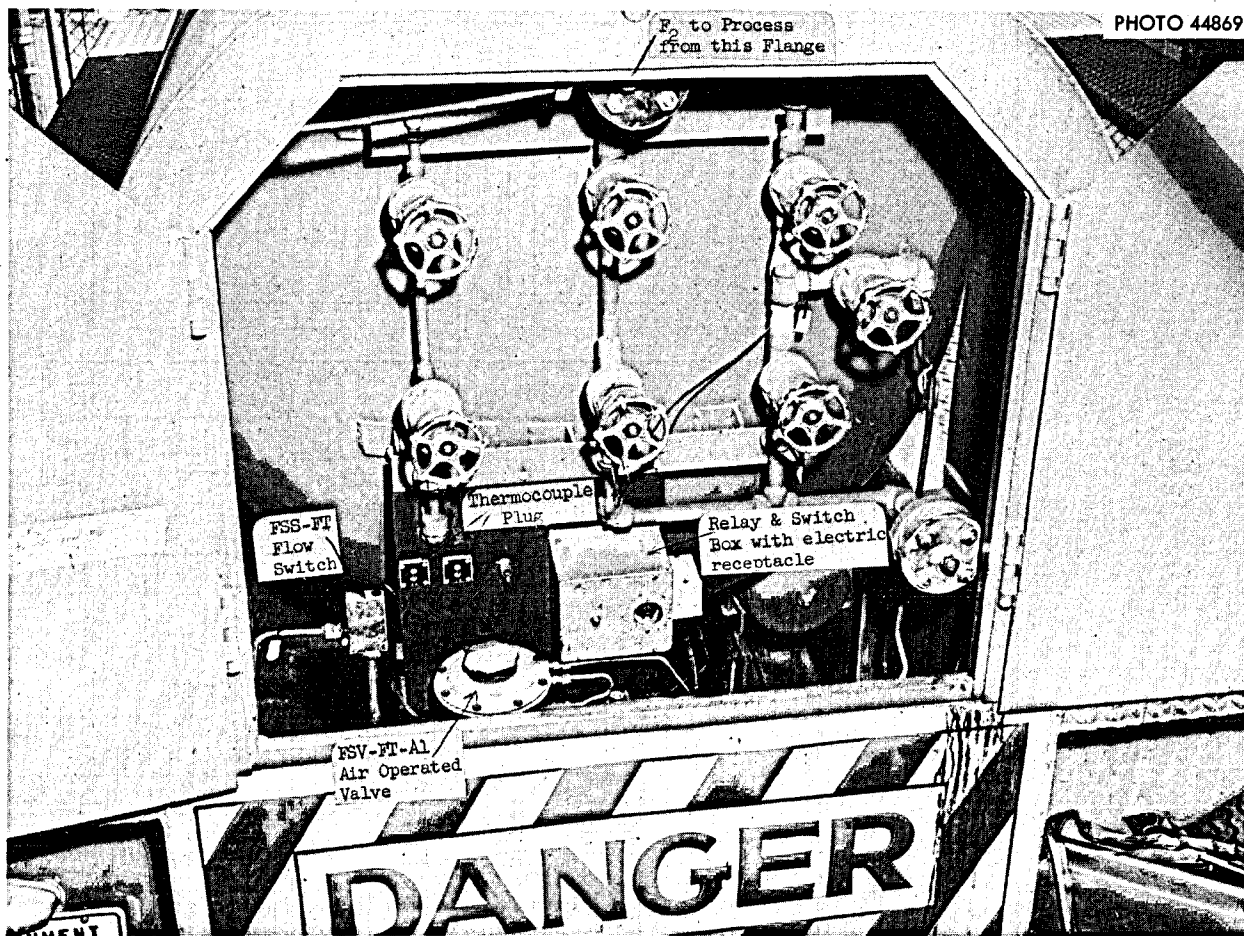
Fig. 3.13.12. Fluorine gas supply tank.
